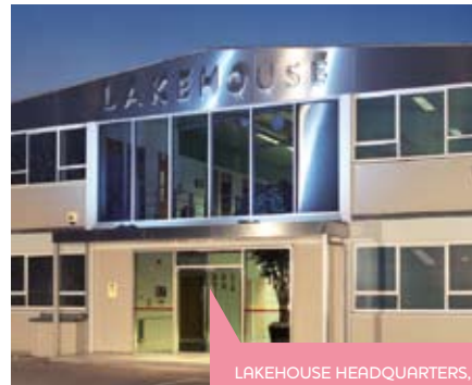
LAKEHOUSE HEADQUARTERS, ROMFORD
